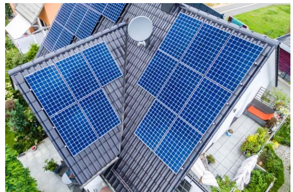
10kWp Neunkirchen am Brand
