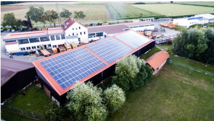
90 kWp Bauhof Eggolsheim - Neuses
